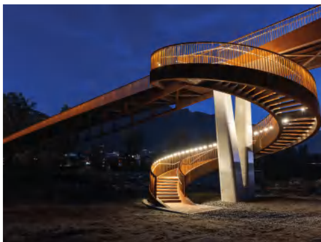
LaneLED WALL, Passerelle de Torretta Bellinzona
