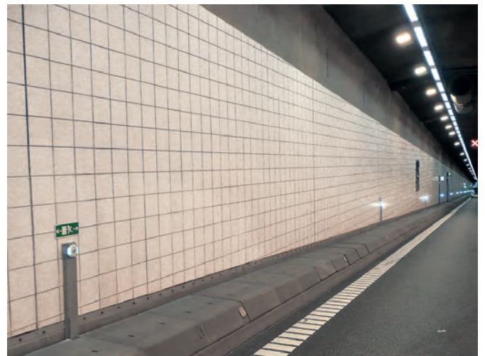
Tunnel Limfjord Danemark
