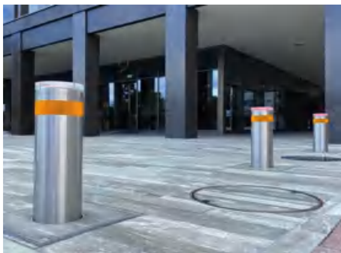
Retractable bollards 2 Schaan
