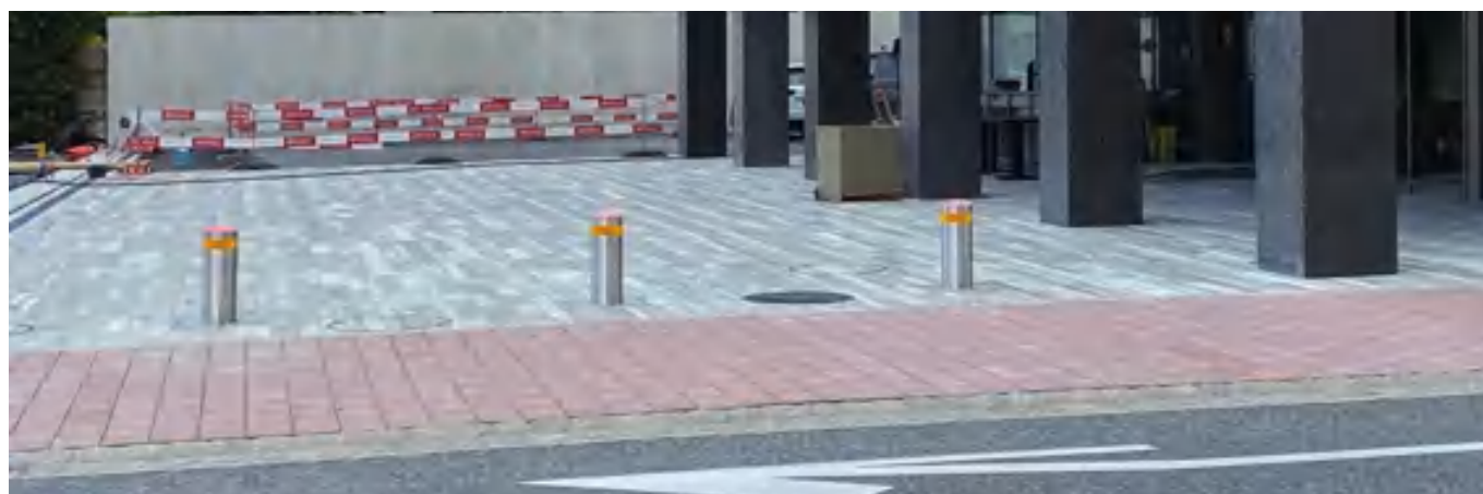
3x Retractable bollards 2, Office building
