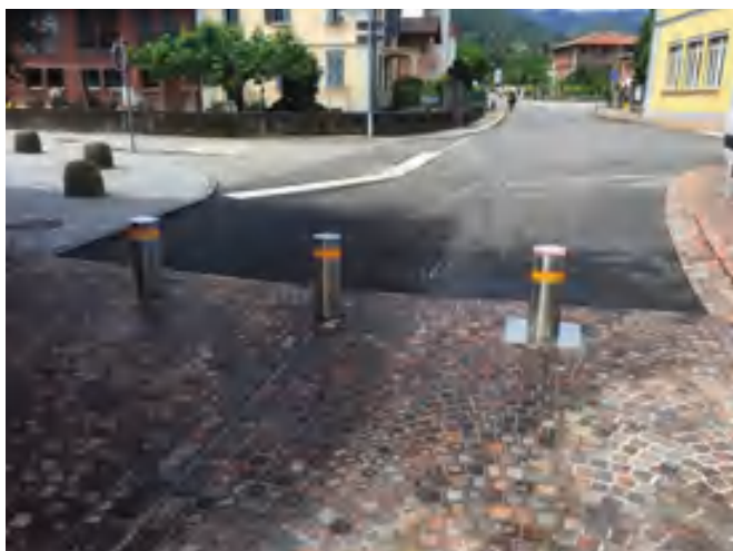
Retractable bollards 2 and fixed bollards Caslano
